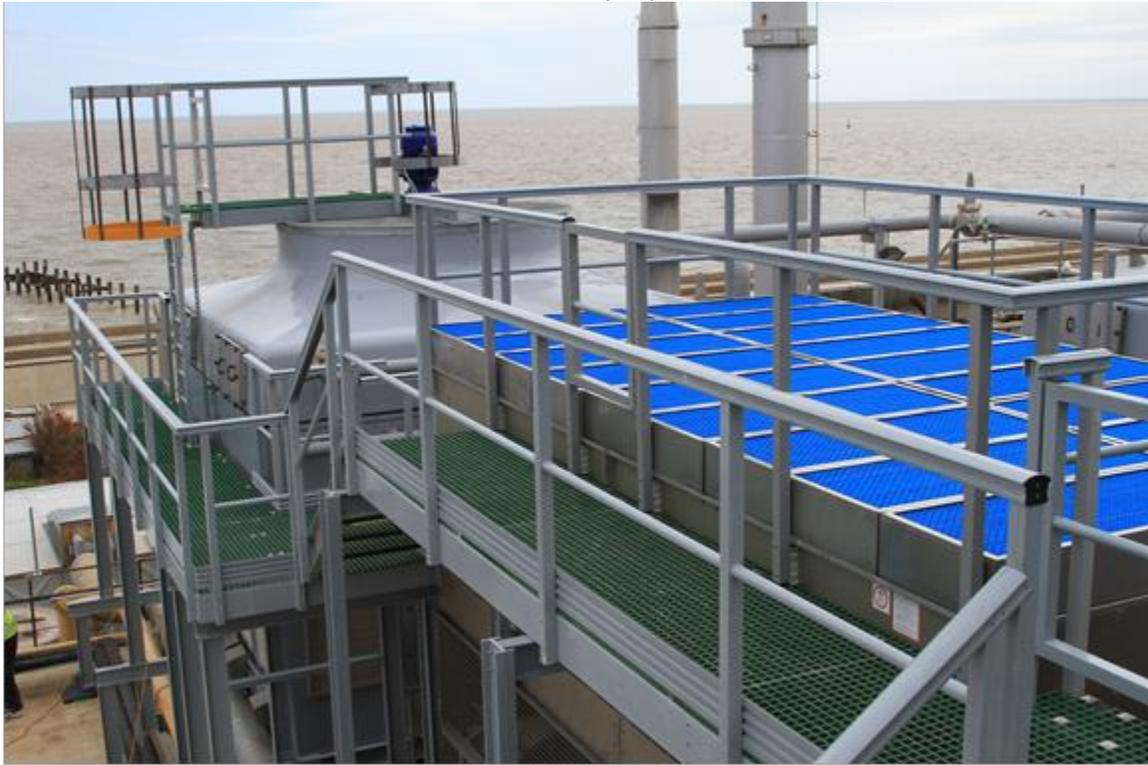
Because the new units are more efficient and more effective, these condensers have become the 'lead machines', and the older condensers will only be used periodically as additional cooling is required.
