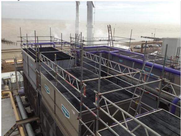
The old evaporative condensers were constructed from coated mild steel and had suffered from severe corrosion. Birds Eye was keen to avoid this on the new installation to keep maintenance and running costs to a minimum and extend the lifespan of the units.
